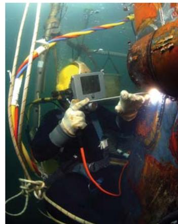
*Commercial divers performing underwater welding or cutting are exposed to burn damage inflicted by sparks and metal spatter*
